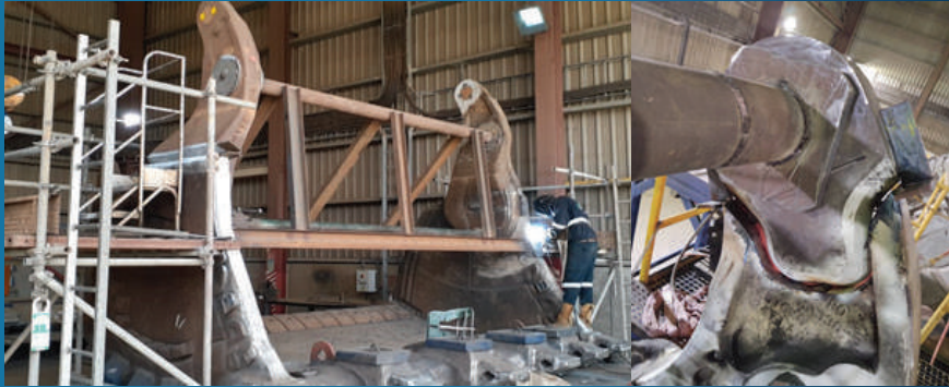
Clam Hinge replacement & repair
