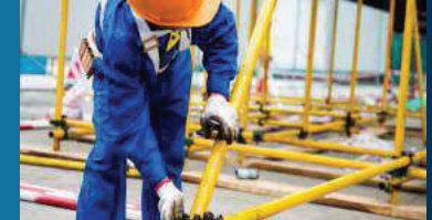
Scaffold Inspection and Erection
